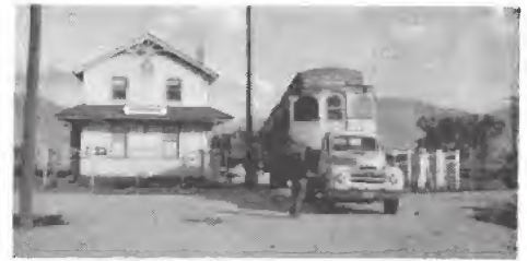
Corinne Railroad Village Museum's recent addition being guided into the Village Yards by Dallas Green. Dale Chirstensen is driving the truck. The coach, an old Bamberger car, was moved recently from Pioneer Village and has now been painted and reroofed and is serving as a museum.
